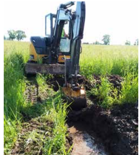
Repairing a tile blowout.
