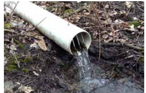
Tile outlet with a rodent guard.
